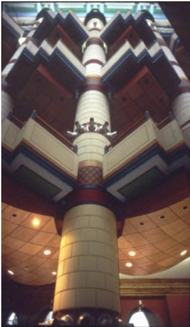
The 'collars of spikes' are A/C efflux cones that can silently fling outlet air some 30 feet. The single protusion in the top quarter is the ceiling uplighter that extends automatically at dusk.
